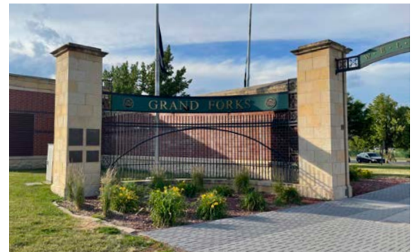
Existing Conditions, Floodwall Gateway at Demers
