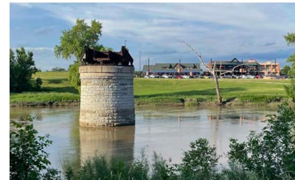
Historic Swing Bridge Foundation in Red River
