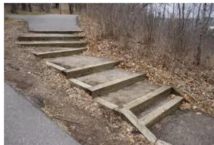
Example of box steps
