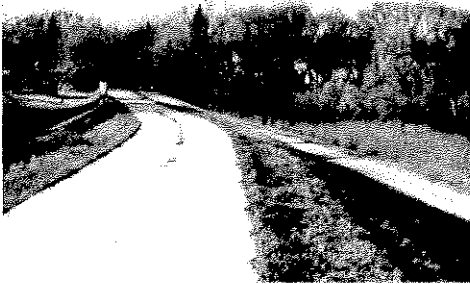
Figure 28: The existing levee trail behind the Grand Forks Chamber of Commerce is the type of trail that is anticipated throughout the Greenway.
